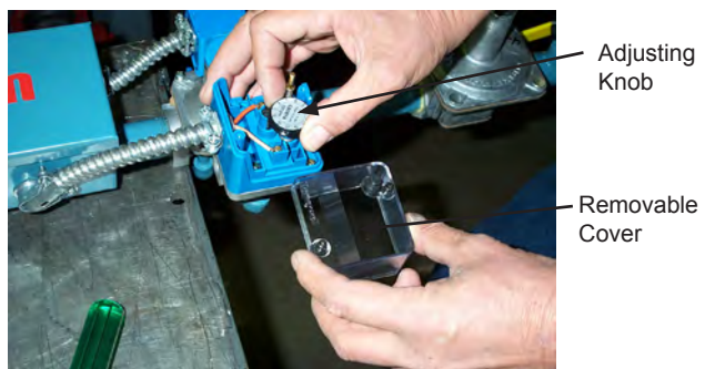
Figure E-8 Gas Pressure Switch Adjustment
